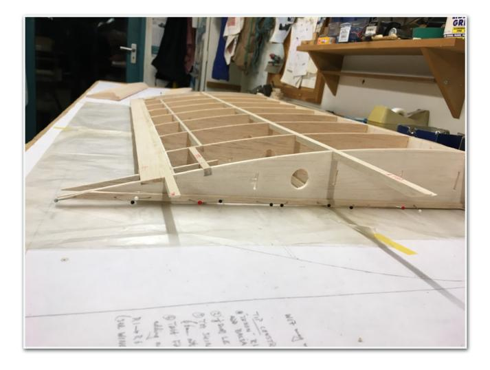
Note jigs for washout and holding end of wing at 90 degrees ( where IS that symbol for degrees ) and at the correct angle for the dihedral at the centre.
