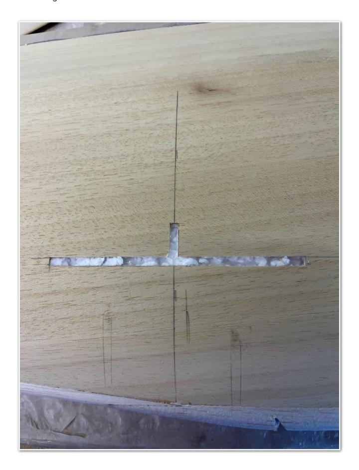
Then formed the slot using my converted soldering iron gun.
